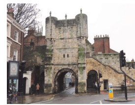
Bootham Bar (with portcullis and walk-through room)
